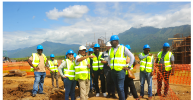
GLDP delegates during a site visit at the KSCL Expansion Project.
