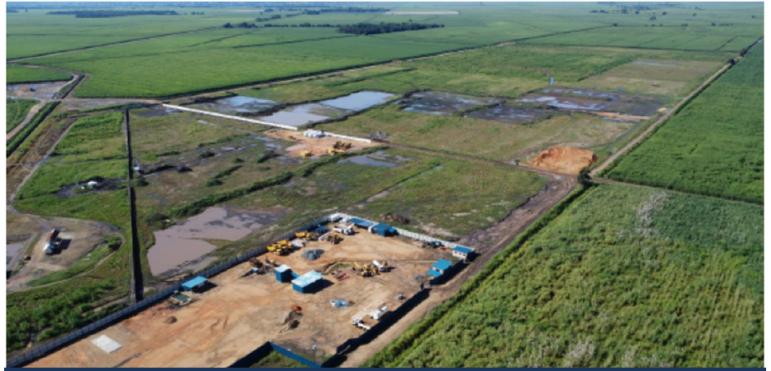
Aerial footage of the K4 Expansion Site
